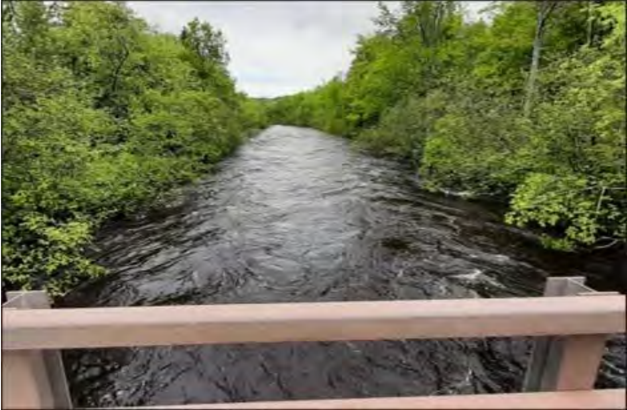
Start of Reach 2 – Downstream of South Drive bridge at 1,200 cfs
