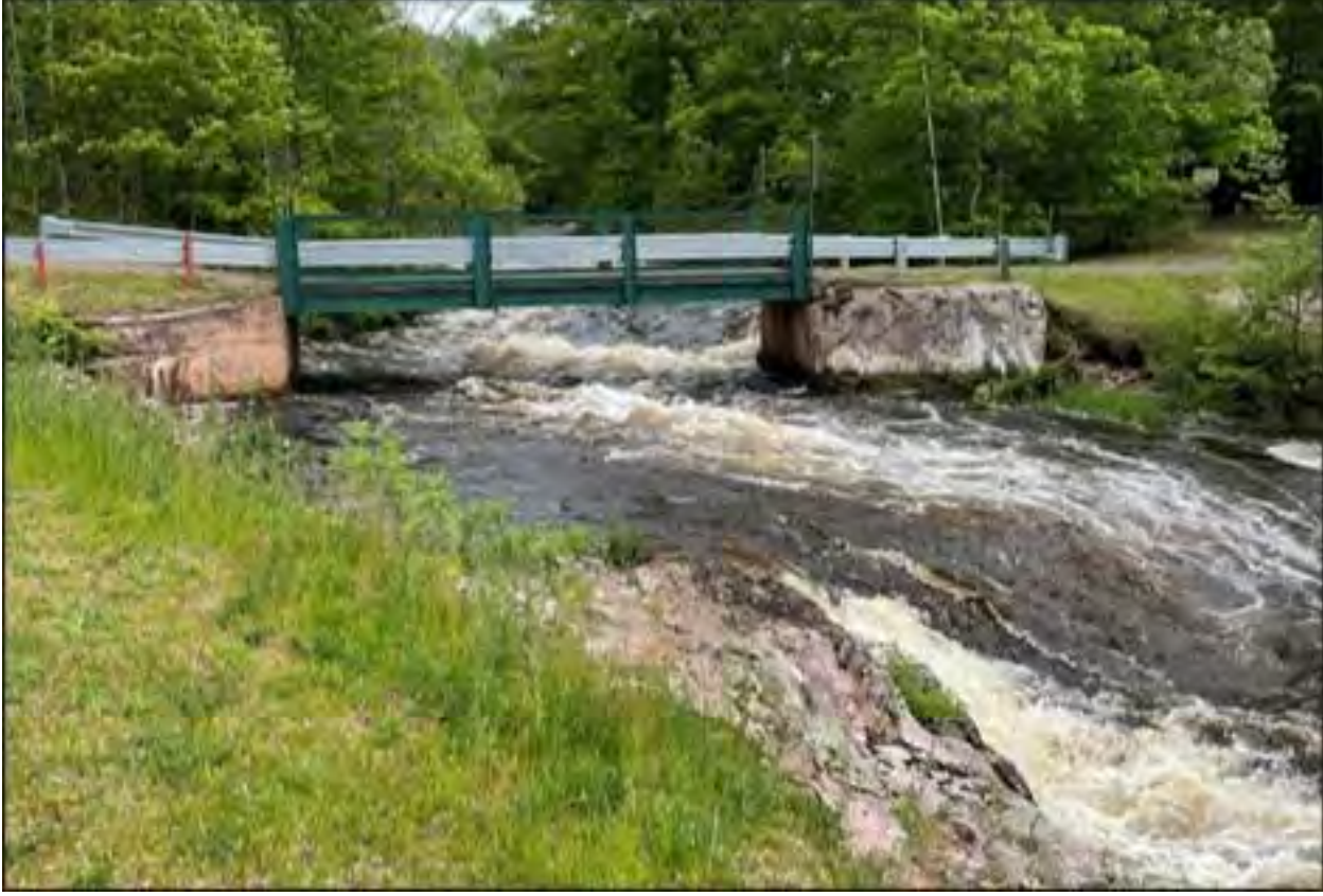
End of Reach 3 – Kimball Town Park bridge downstream of Kimball Falls at 1,200 cfs
