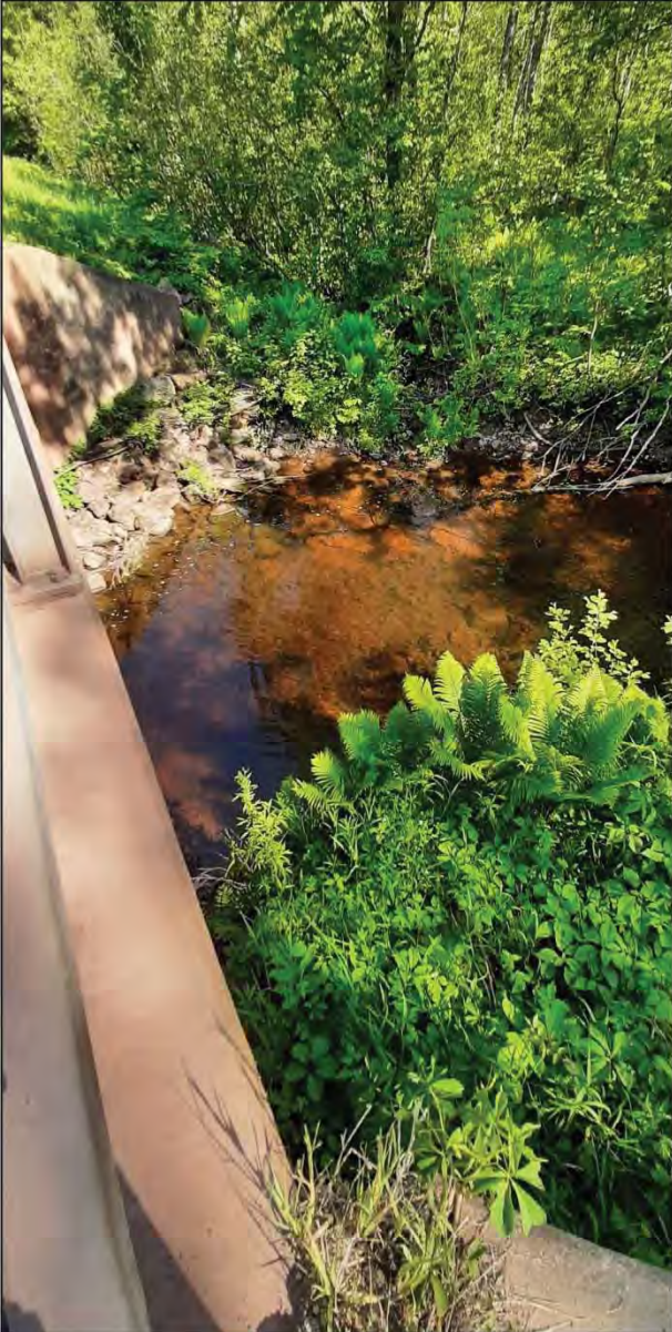
Boomer Creek Upstream from Bridge Photo 8
