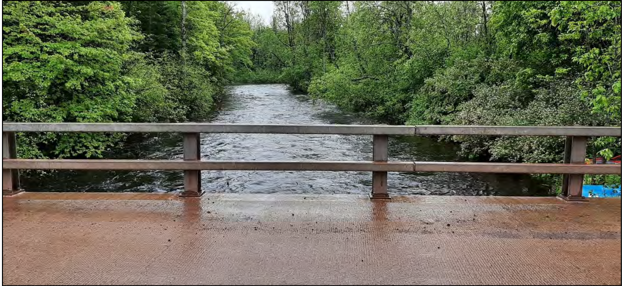
End of Reach 1 – Upstream of South Drive bridge at 600 cfs
