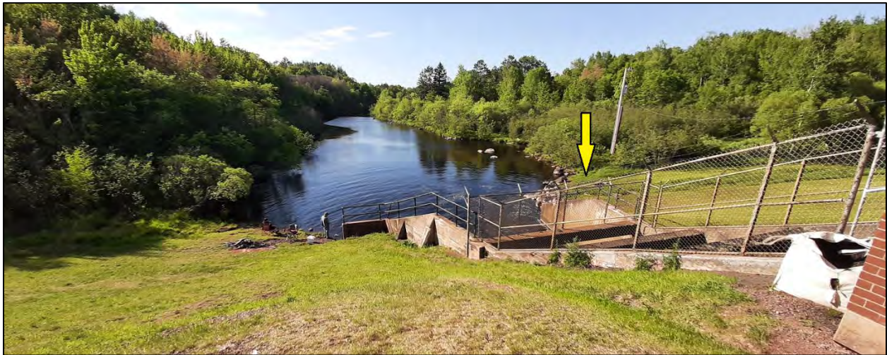
Figure 4.2.2.1-1 Put-In Location and Access at Gile Dam
