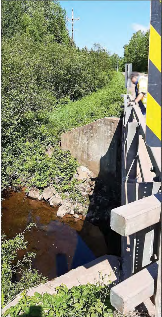
Boomer Creek Downstream from Bridge Photo 9
