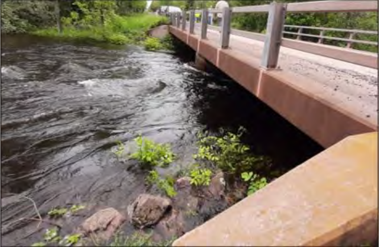
End of Reach 1 – Upstream of South Drive bridge at 1,200 cfs, clearance roughly 3 feet
