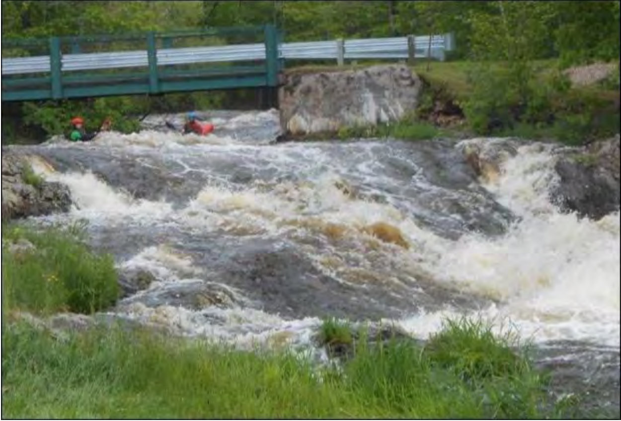
End of Reach 3 – Boaters under Kimball Town Park bridge at 1,200 cfs
